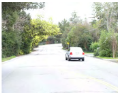
This segment of Santa Cruz Avenue (just west of Avy) is wide enough to comfortably accommodate a Class III facility. The route would serve as a connection to Sand Hill Road and Alpine Road.
