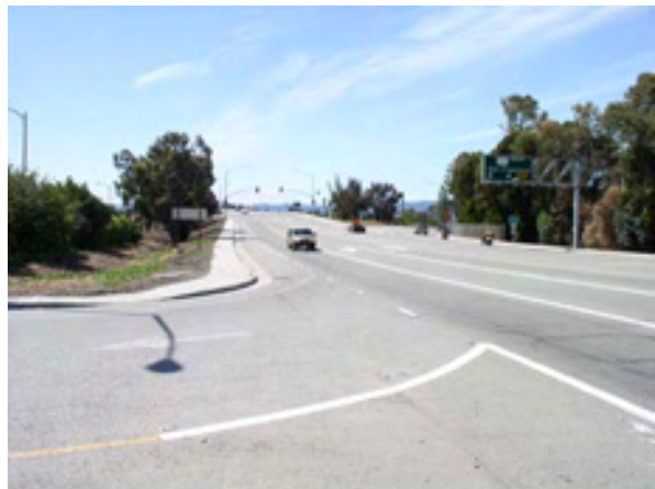
Marsh Road provides an important crossing of U.S. 101 and a direct connection to Bayfront Park and the Bayfront bike path, but crossing the interchange requires cyclists to merge across several free turn lanes.
