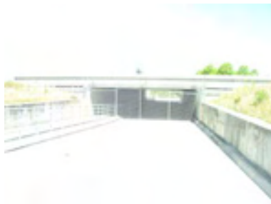
The existing undercrossing is currently fenced off. Safety and security improvements such as lighting would be required prior to using it as a bicycle/pedestrian facility.
