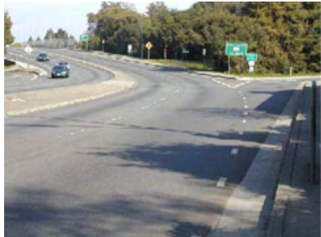
The U.S. 101 interchange at Willow presents a difficult crossing for less experienced cyclists due to the lack of a designated bike lane and high-speed free turn lanes on and off the freeway
