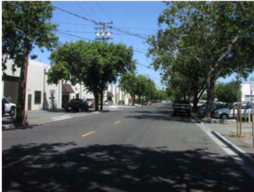
O'Brien Drive provides a direct connection between Menlo Park and East Palo Alto on the east side of US-101; a bike lane striping plan for this roadway has already been completed by the City of Menlo Park.
