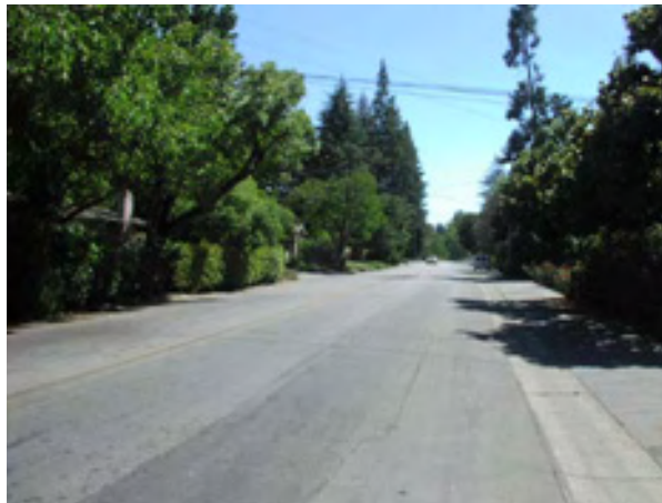
The Oak Class III neighborhood route would provide a continuation of the Middle Avenue facility, extending to Sand Hill Road.
