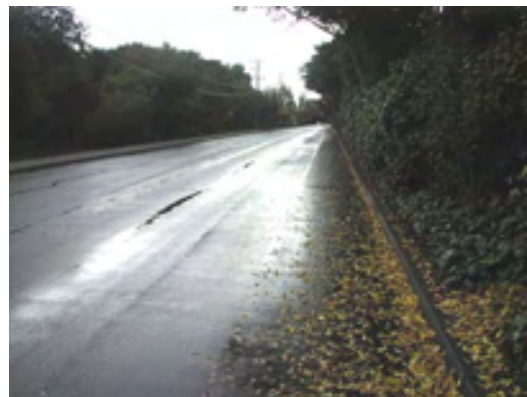
Class II bike lanes on Bay Road lack signage and need re-striping and stenciling. Following a rainstorm the bike lane was covered with wet leaves in many places.
