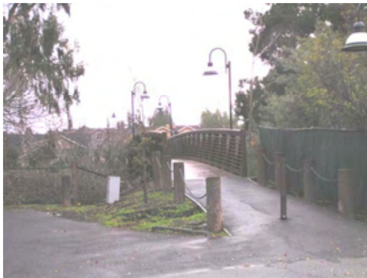
The San Mateo Drive bicycle and pedestrian bridge provides an important connection between the City of Menlo Park and the City of Palo Alto.
