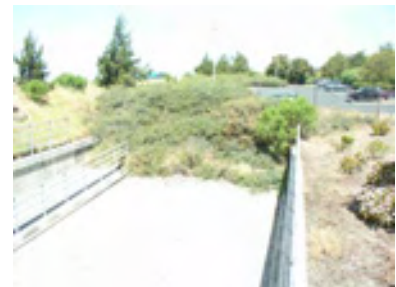
The existing entry ramp on the east side of Bayfront Expressway is blocked by the Sun Microsystems parking lot. A new ramp would need to be provided to meet ADA standards.
