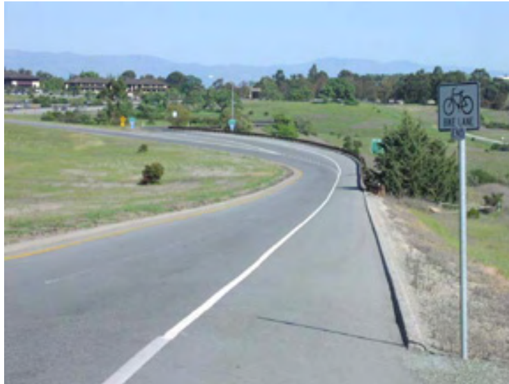
The bike lane on Sand Hill Road eastbound currently terminates prior to the I-280 interchange. In the westbound direction, bike lane striping has been carried through the interchange to improve conditions for cyclists on this heavily-used bicycle route.
