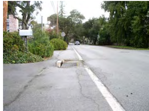
This drainage gate, in the Encinal Avenue bike lane at the intersection with Laurel Street, forces cyclists to veer into the travel lane to avoid it.
