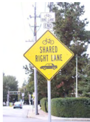
The “Shared Right Lane” sign on EB Ravenswood Avenue was installed to enhance the safety of bicyclists approaching the Caltrain railroad crossing where the bike lanes end and the auto lanes merge.
