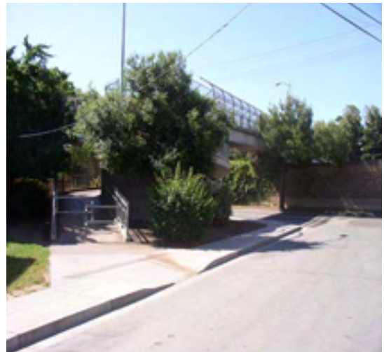
The existing Ringwood Avenue crossing has security issues related to the design of the bridge and lack of visibility due to overgrown vegetation.
