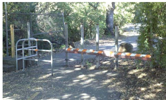
Gunn High School Path at the terminus of Los Robles Avenue. This barrier design is typical of many existing trail intersections, and complicates use by people with disabilities, strollers, and bicycles with trailers.
