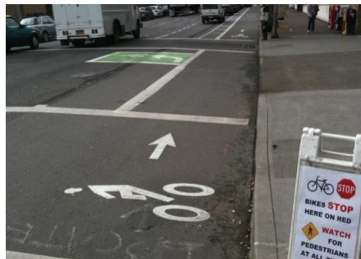
Bike box positions bicyclists to make a left turn from a cycle track in Portland, OR.
