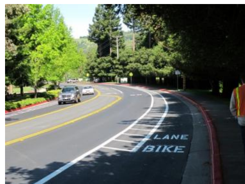
Fairfax, CA: Buffered bike lanes installed as part of a Safe Routes to School project on Sir Francis Drake Blvd (arterial).
