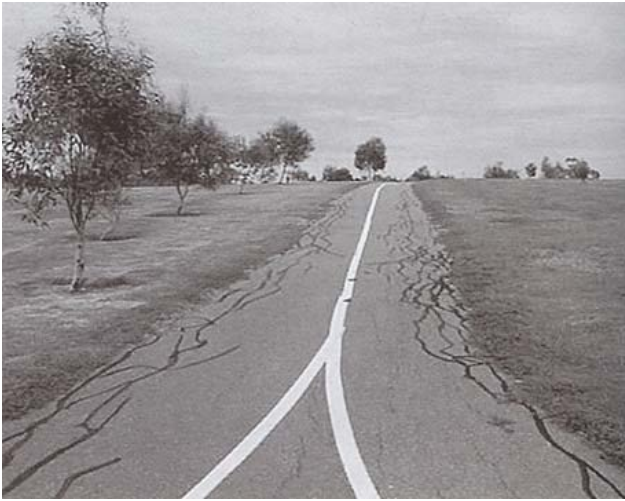
Figure E 1: Asphalt paths requiring maintenance
