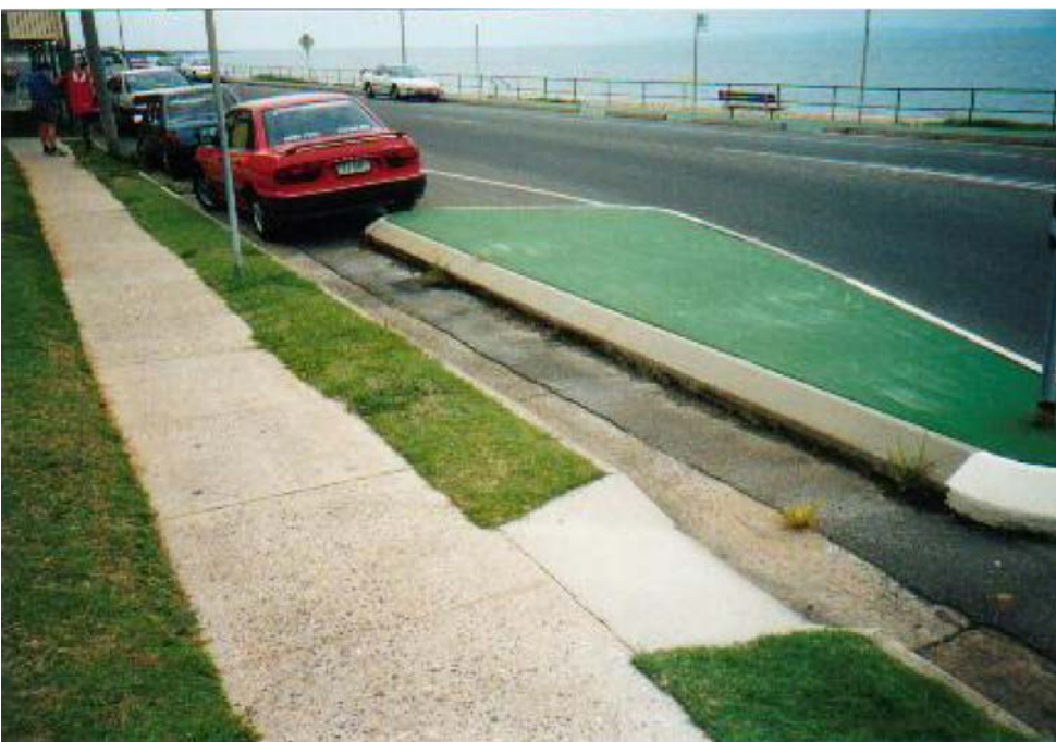
Figure 4.12: Parked vehicle blocks cycle bypass
