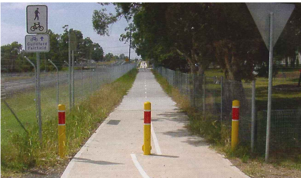
Figure 7.17: Example of a bollard treatment
