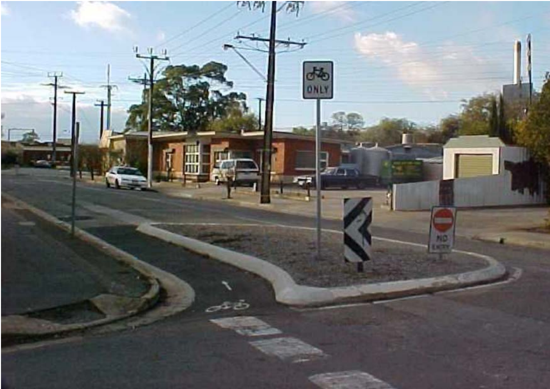
Figure 4.13: Cycle bypass at half road closure
