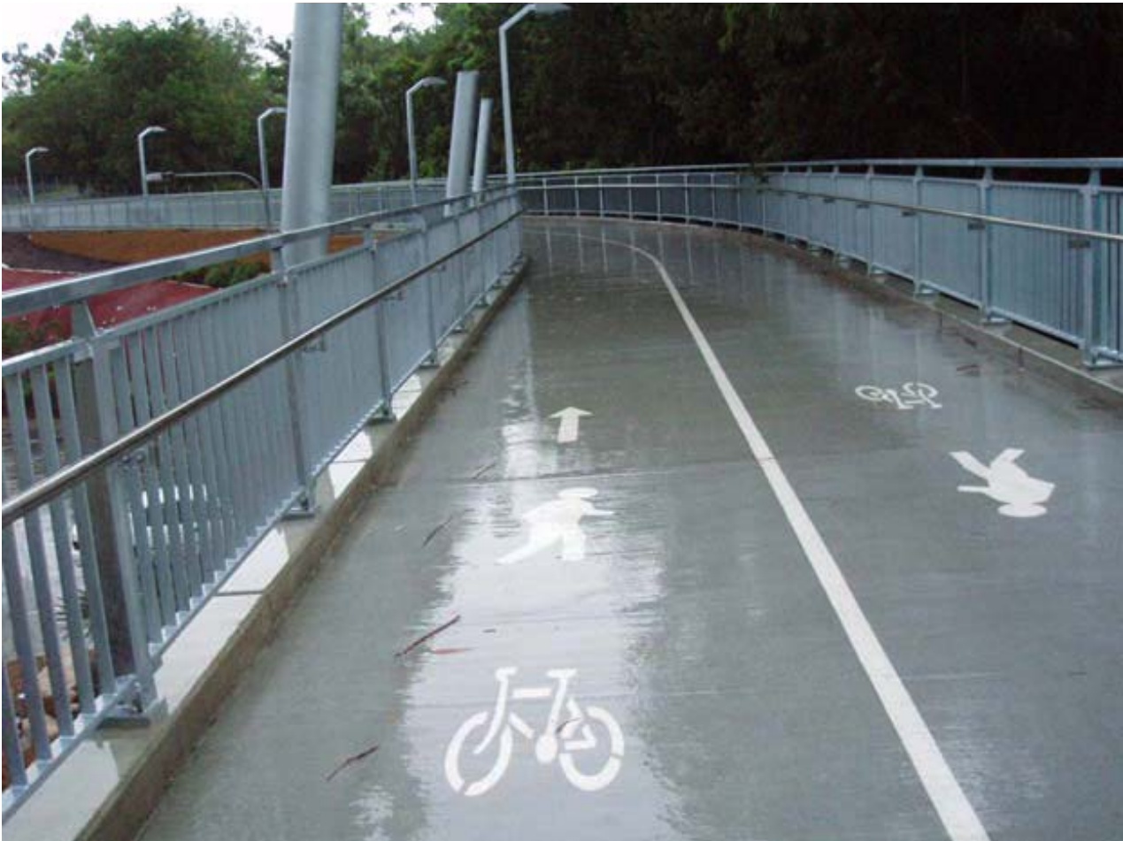
Figure E 7: Concrete path (Normanby Pedestrian and Cycle Link, QLD)
