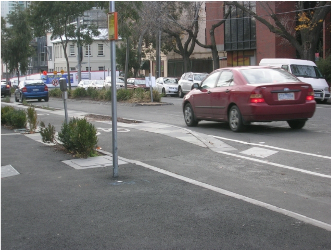
Figure 4.7: Kerb separated bicycle lane
