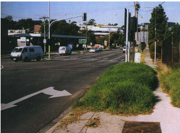
Figure G 1: The path to pedestrian signals is narrow and overgrown
