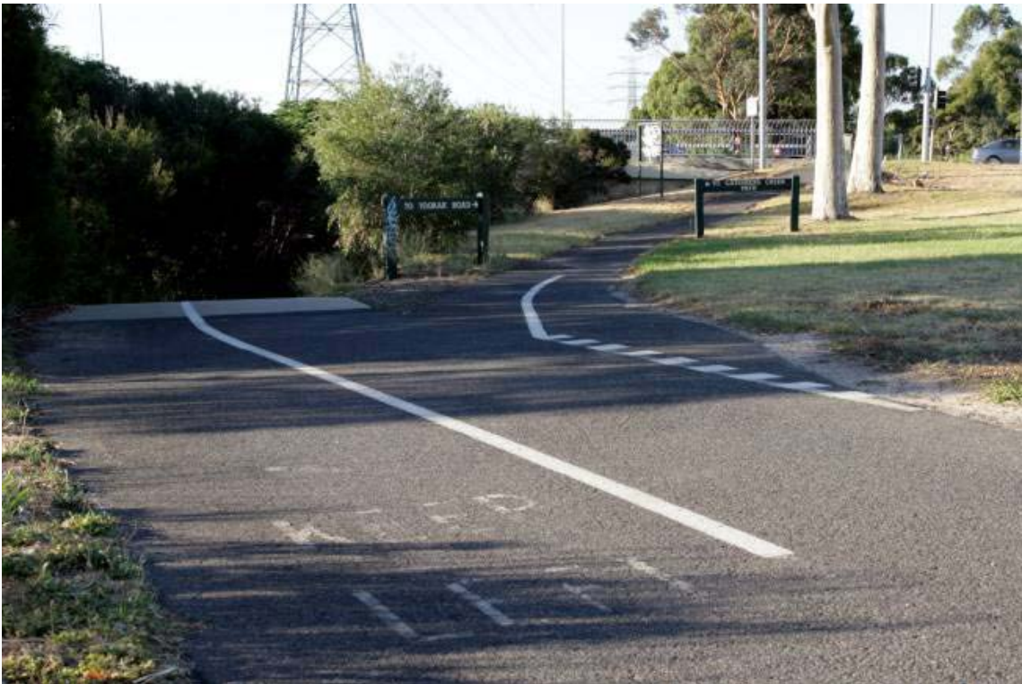
Figure G 2: The link path from Toorak Road joins at an acute angle, with restricted sight distance
